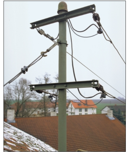
Service entry through overhead system
